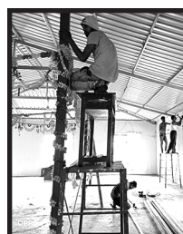
Staff Room Overroof
