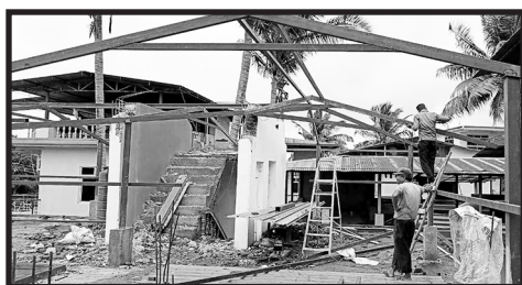
Demolition - Staff Work Areas Etc.
