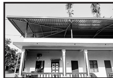
Staff Room Overroof Finished!
