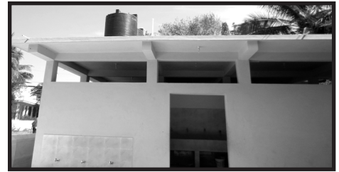
New Washroom, Bathroom, Shower Facility
