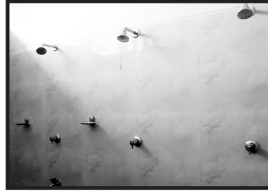
Part of Large Shower/Washing Area
