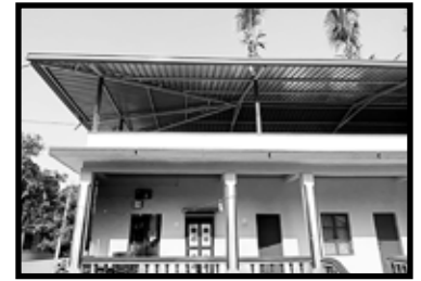
Staff Room Overroof Finished!
