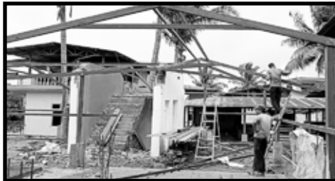
Demolition - Staff Work Areas Etc.
