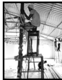
Staff Room Overroof
