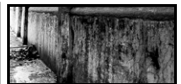
Old Low Moldy School Wall
