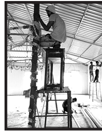
Staff Room Overroof
