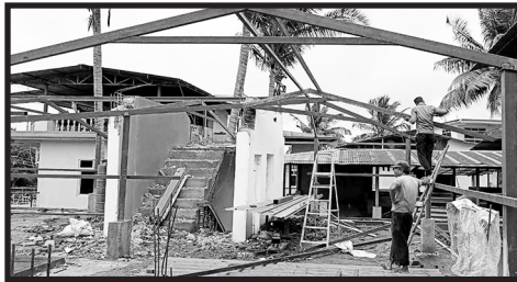
Demolition - Staff Work Areas Etc.
