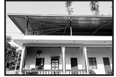
Staff Room Overroof Finished!
