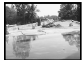
Repair Starting on School Roofs
