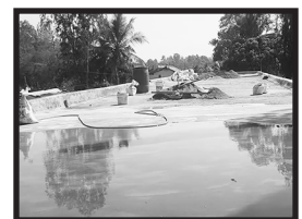
Repair Starting on School Roofs
