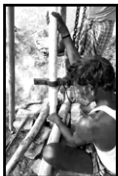
Water Pipes Replaced
