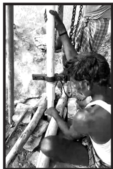
Water Pipes Replaced
