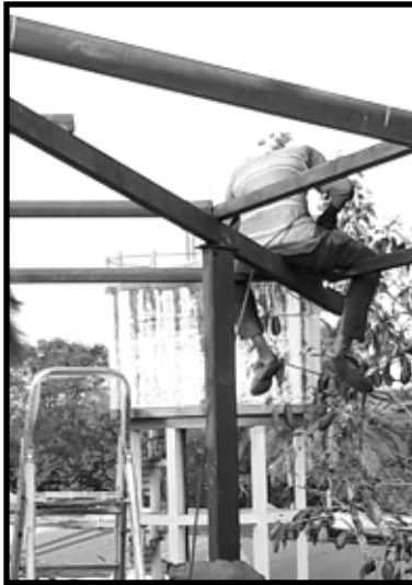
A Small Piece of the Decaying Roof, Workers Doing Repairs and Beginning the Over-Roof Supports
