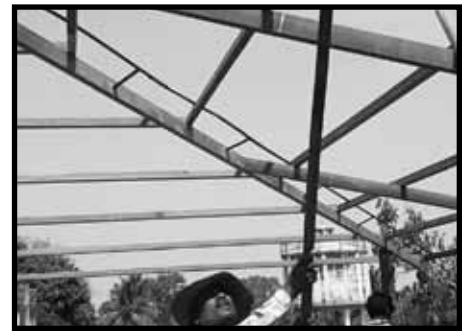
Over-roof Under Construction, OPH
