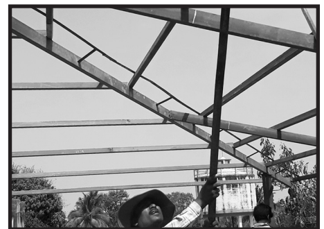
Over-roof Under Construction, OPH
