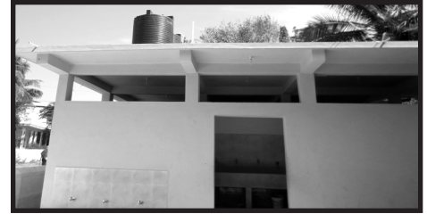
New Washroom, Bathroom, Shower Facility
